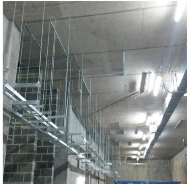
Figure 1: Unistrut channel support system
